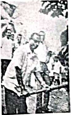
CONSTRUCTION OF A ROAD
