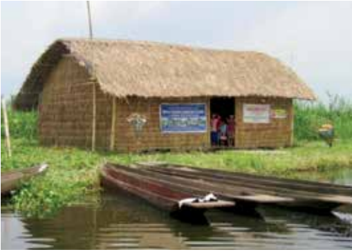
Figure 3: The Loktak Floating Elementary School in Manipur is built with material like bamboo and thatch.
