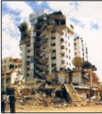
Fig. 3.3a: Destruction caused by an Earthquake in Gujarat
