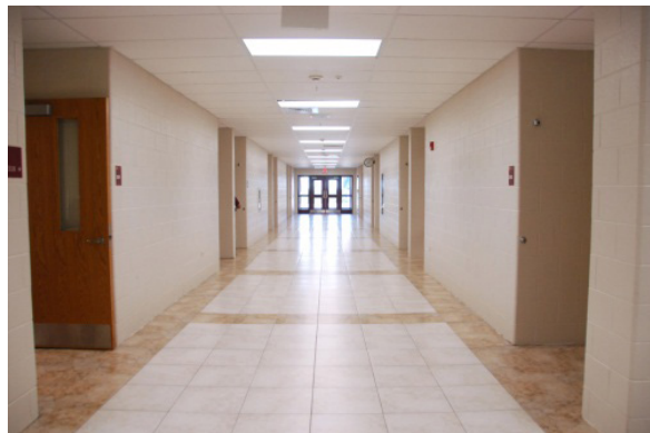
“Cells and bells:” double-loaded school corridor with concrete block walls
