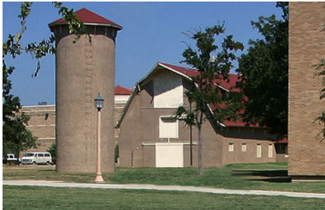
The Texas Technological College Dairy Barn was used as an agricultural teaching facility until 1967.
