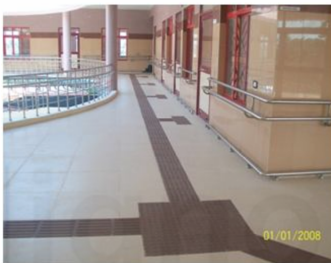
Figure: Indication of the entrance of the classroom and junction point with dot-embossed tiles
