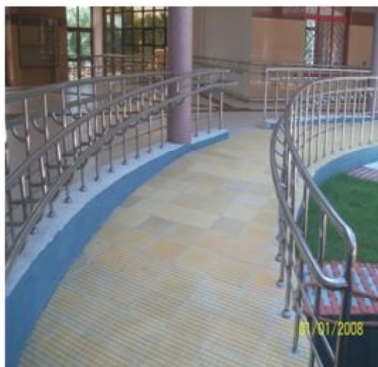
Figure: Ramps with handrails
