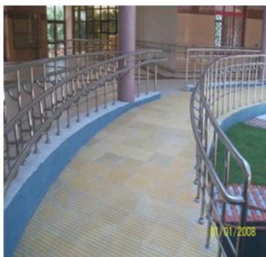
Figure: Ramps with handrails
