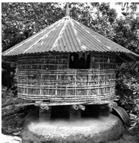
Figure 5: Dhaner Gola , the structure where raw rice is stored
