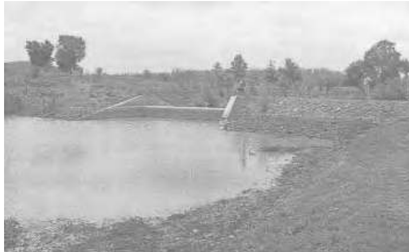
A small dam
